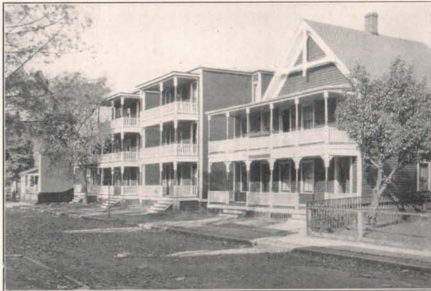
DEPARTMENT OF HOUSING HOUSING PROPERTIES FROM 138 TO 156 QUINCY ST.
